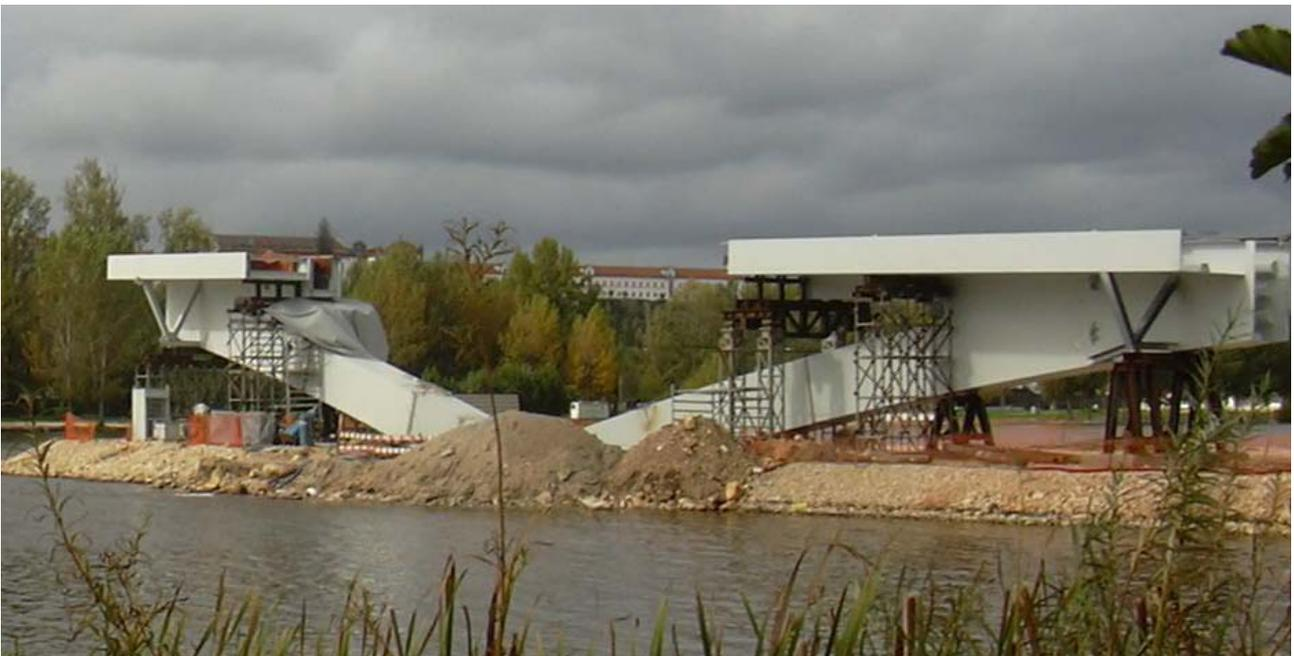
*Fig. 6 – Details of propping of the bridge under construction (October 2005).*
